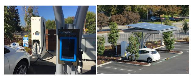
The solar roof has15 modules with a capacity of 4.1kW, providing an estimated yearly production of 7,300 kWh at this location in Santa Clara. This ETM<sup>™</sup> is equipped with the Ideal Power IBC-30kW-480 bi-directional converter with a 30KW capacity to convert AC to DC and DC to AC.
